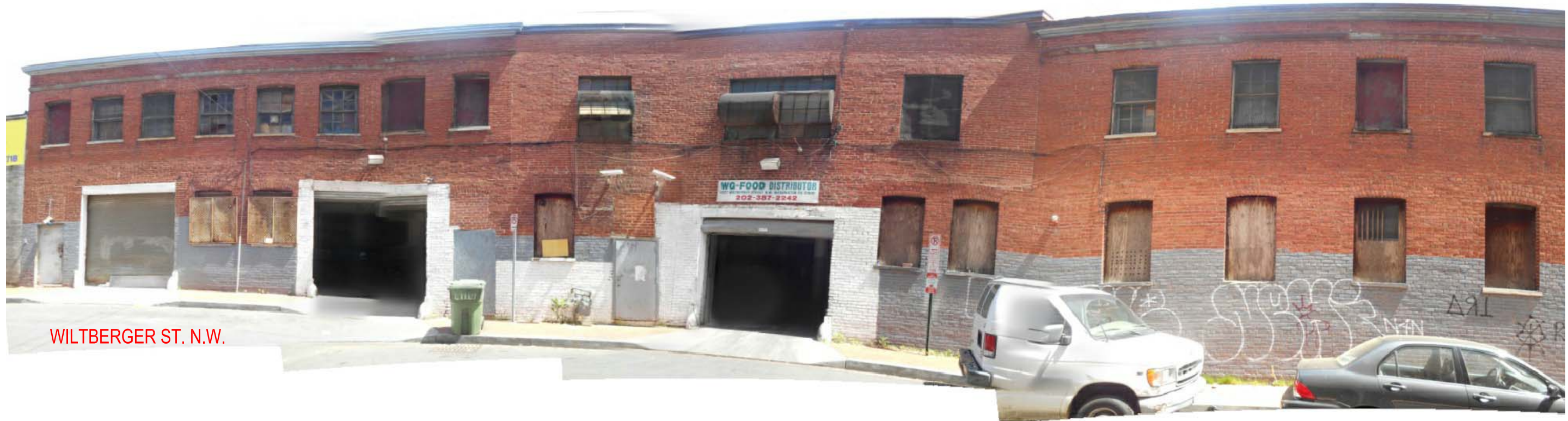
3 - WEST FACADE PANORAMA
