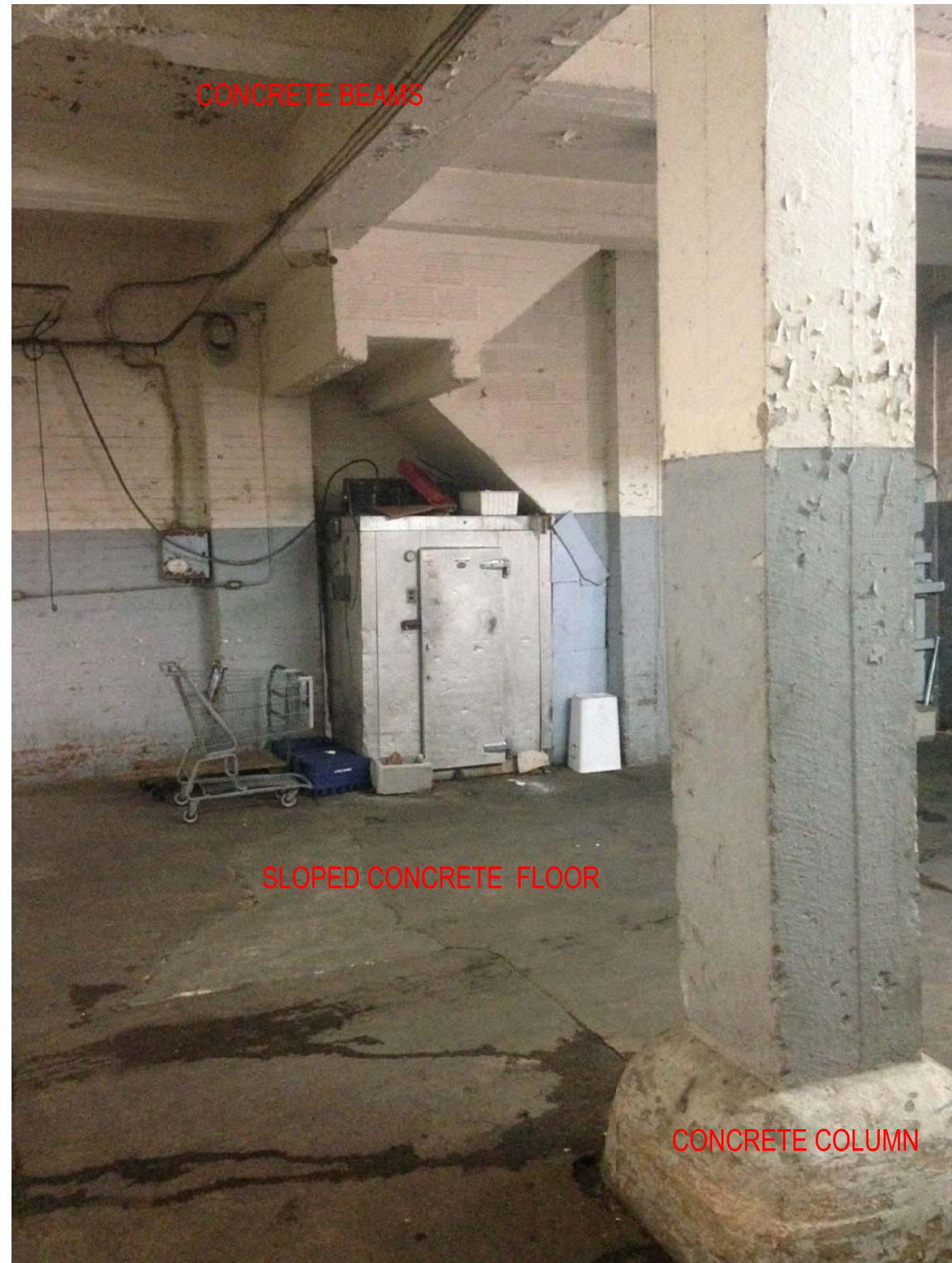
20 - CONCRETE STRUCTURE - FIRST FLOOR
