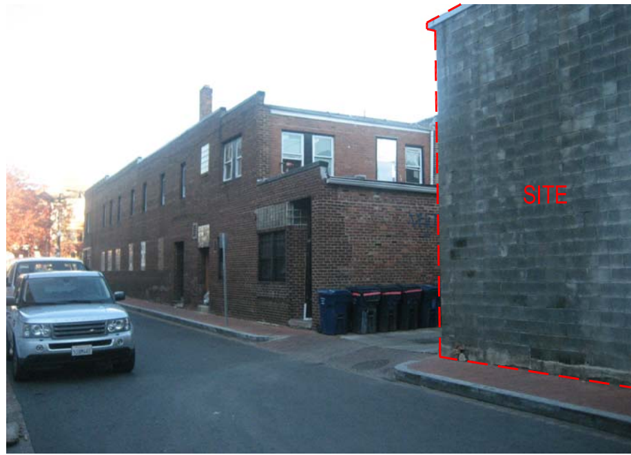
8 - NON-HISTORIC CMU WALL AND NEIGHBORING BUILDINGS
