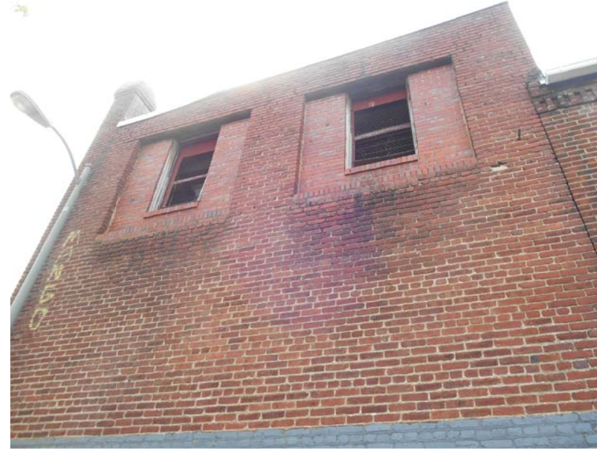
5 - SEMI-INFILLED HISTORIC WINDOWS - EAST FACADE
