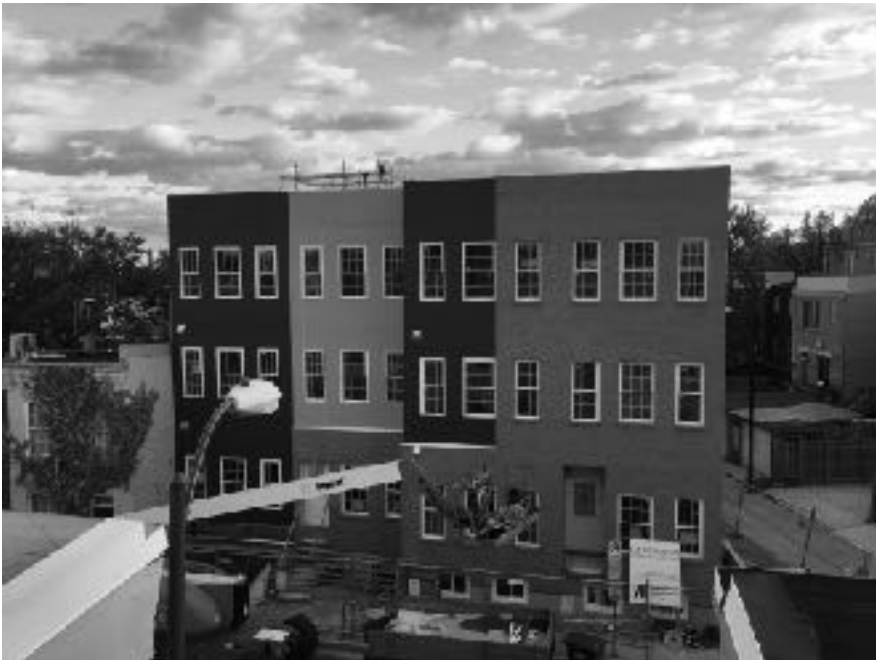
October 22, 2016: Structure spanning 410 and 412 Richardson Place NW. Permit board not erected.
