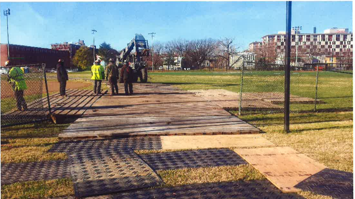
Picture 2: Installation photo showing wooden crane mats.
