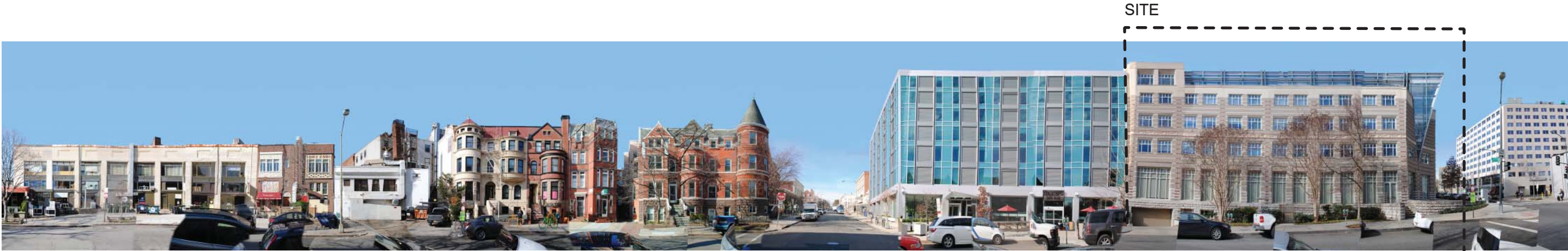
20TH STREET LOOKING WEST
