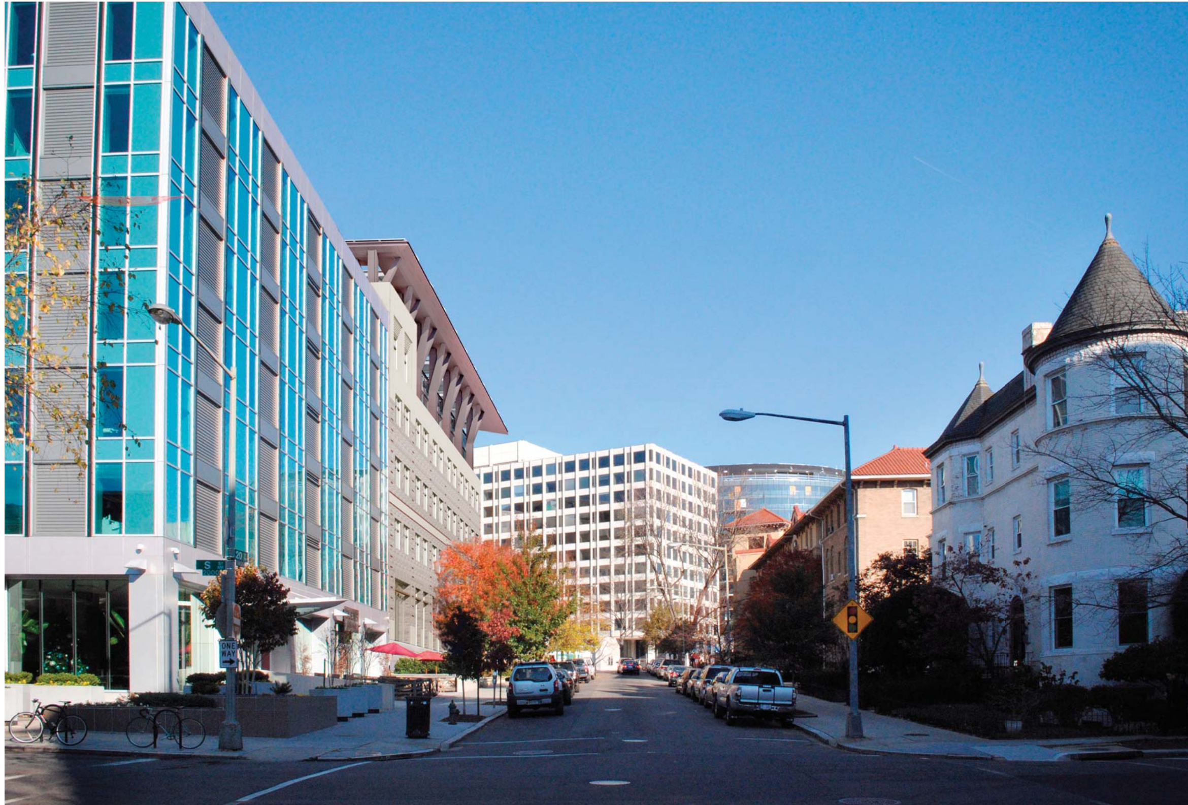
VIEW FROM INTERSECTION OF 20TH & S STREETS NW
