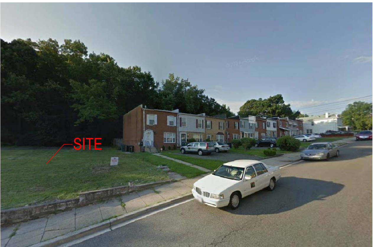
VIEW SOUTH WEST
