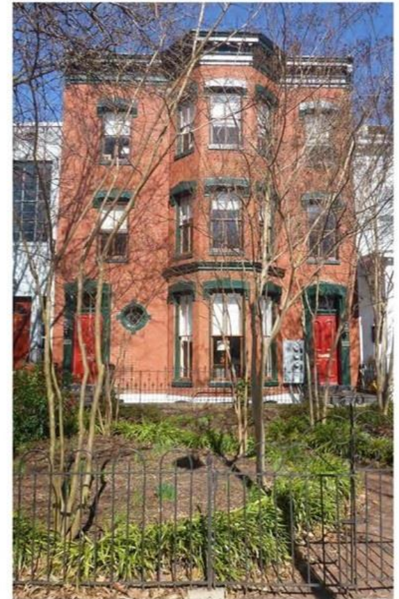
Photo1: View of Existing Front South facade
