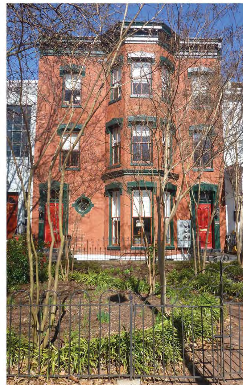
Photo1: View of Existing Front South facade
