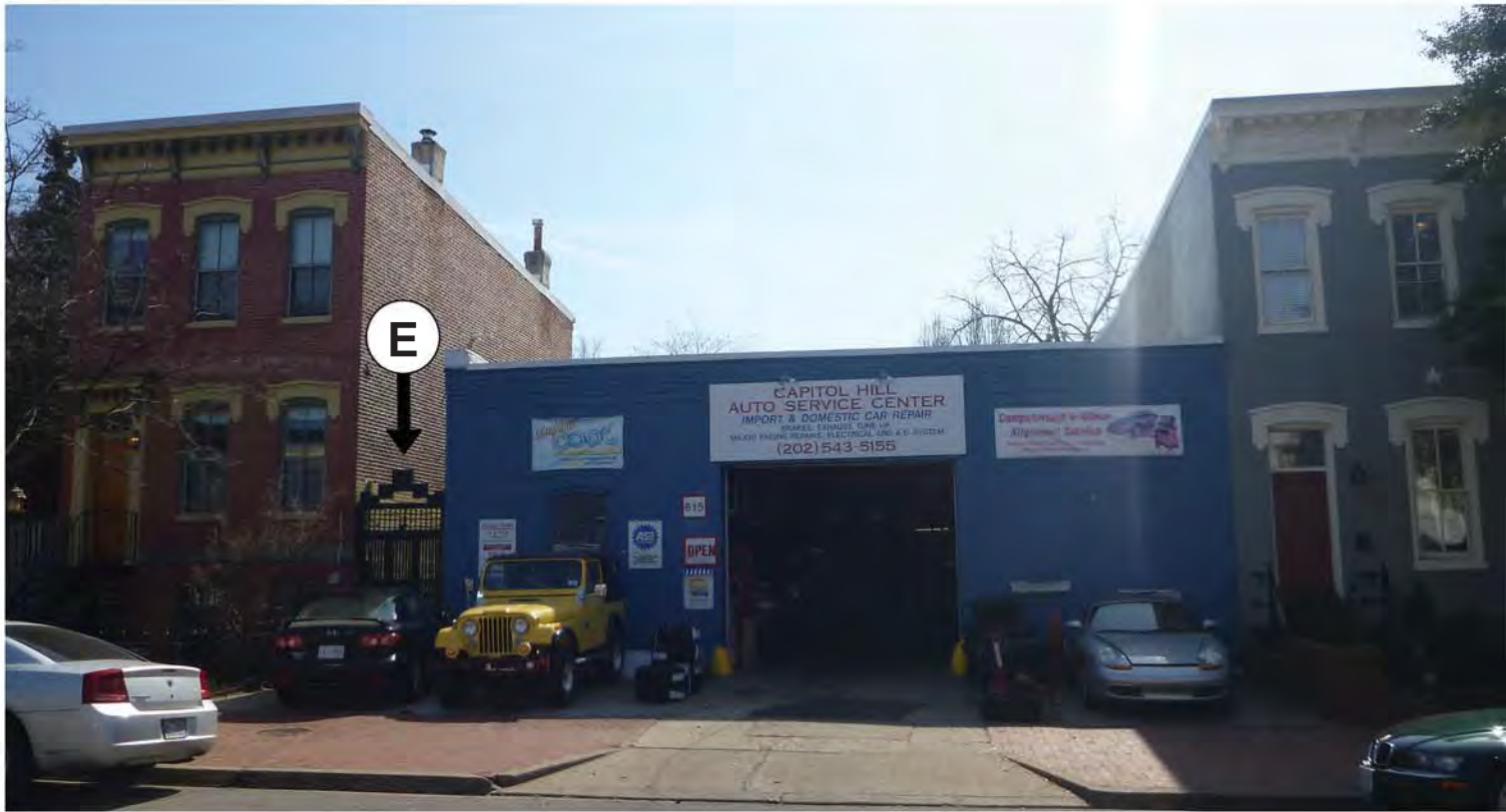
Photo 4: View looking South (Entrance to rear yard noted with an E)
