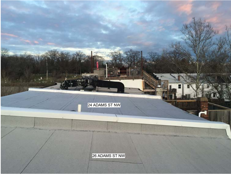
EXISTING ROOF PHOTOS
