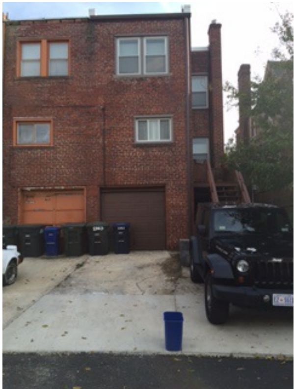
REAR VIEW FROM ALLEY
