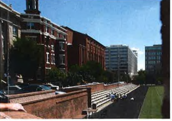
10. WEST SIDE DRIVE AISLE - LOOKING EAST
