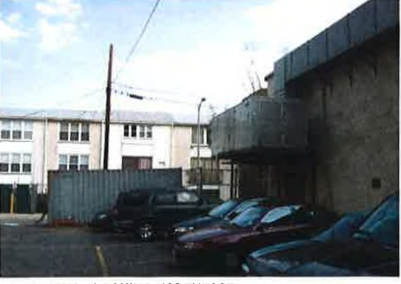
14. PARKING - LOOKING NORTHEAST
