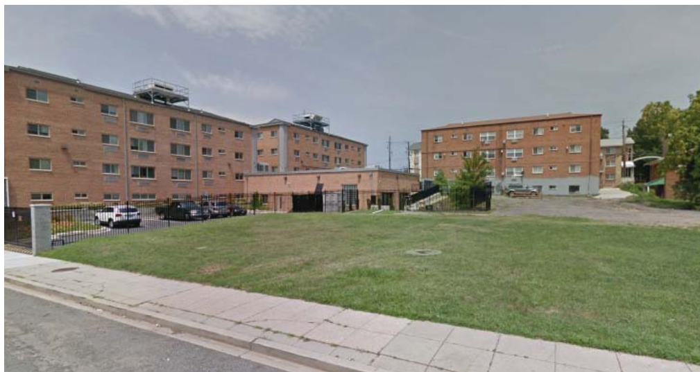
5. Site, Looking Northwest
