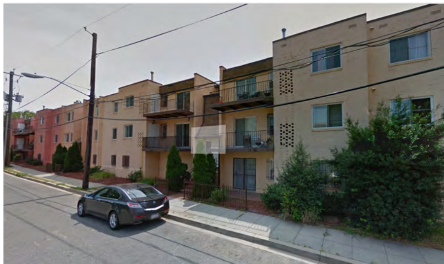
3. D Street, Looking East (Opposite Site)
