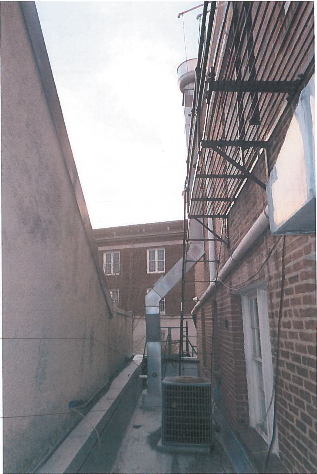
PHOTO SHOWING THE CURRENT CONDITION AT THE FIRST FLOOR ROOF TERRACE OF 1832 WISCONSIN AVE
