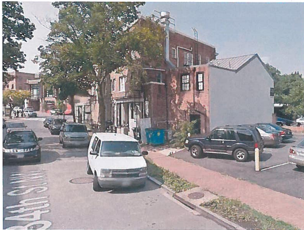
VIEW FROM 34TH ST. SOUTH
