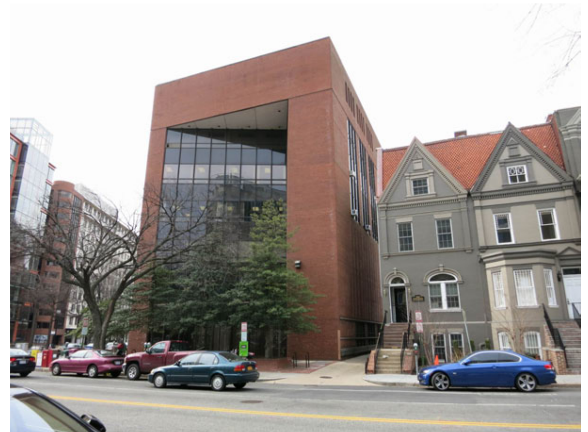
6. EAST ELEVATION, VIEW ALONG 17TH ST. NW
