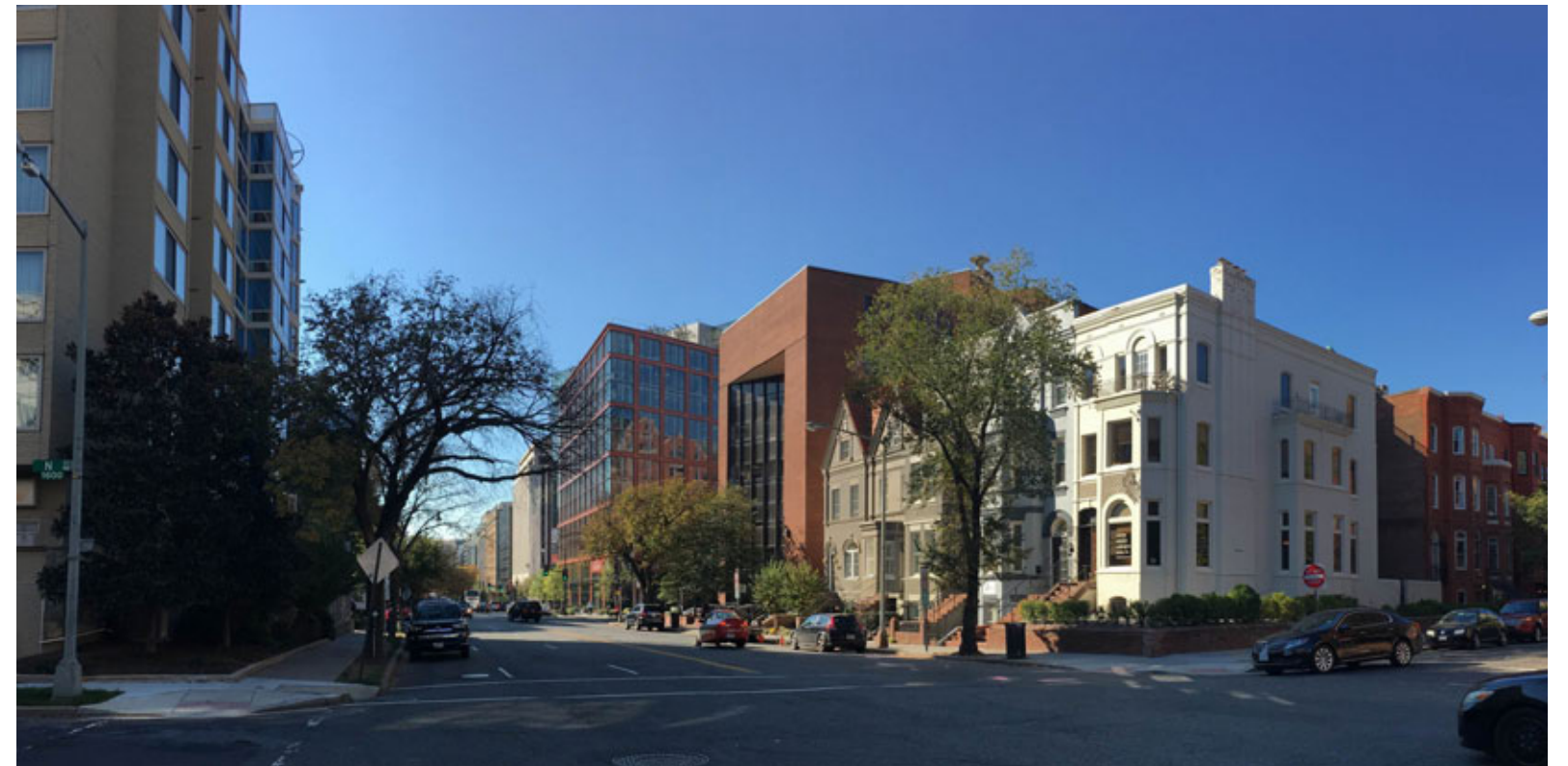
4. VIEW LOOKING SOUTH, DOWN 17TH ST. NW
