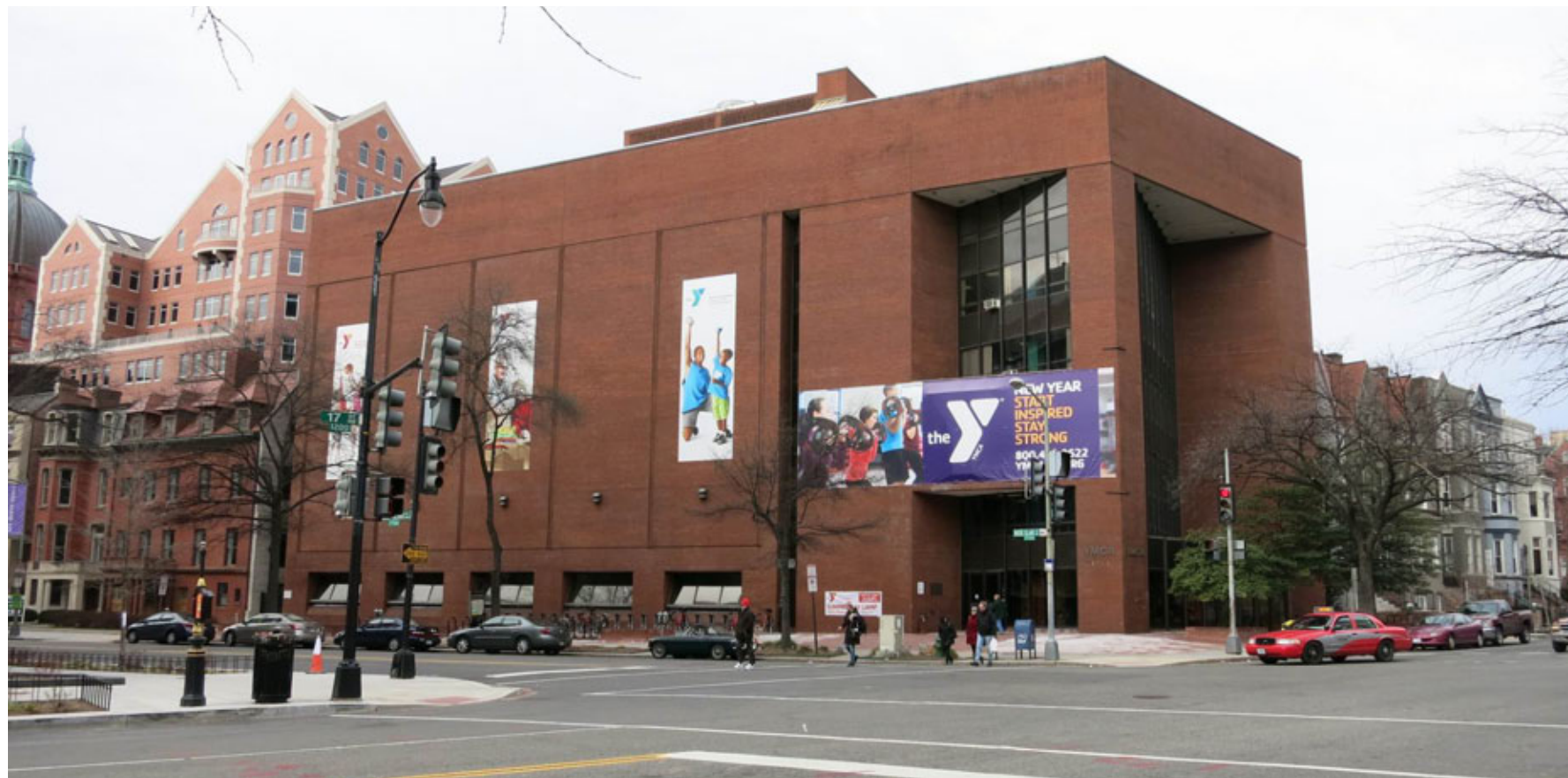
5. SOUTH ELEVATION, VIEW ALONG RHODE ISLAND AVE. NW
