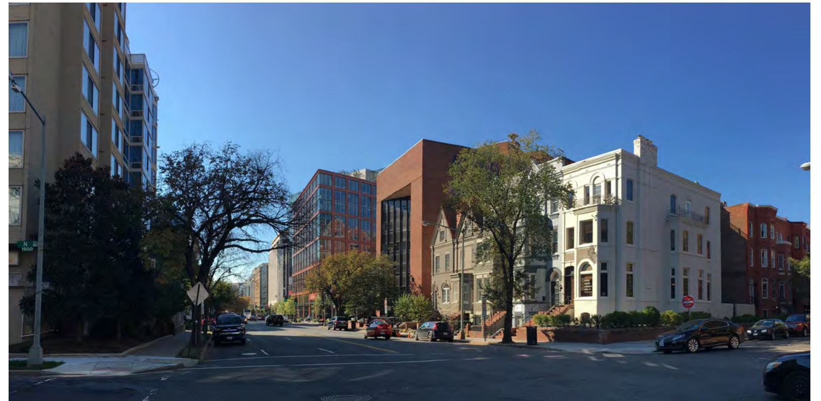
4. VIEW LOOKING SOUTH, DOWN 17TH ST. NW
