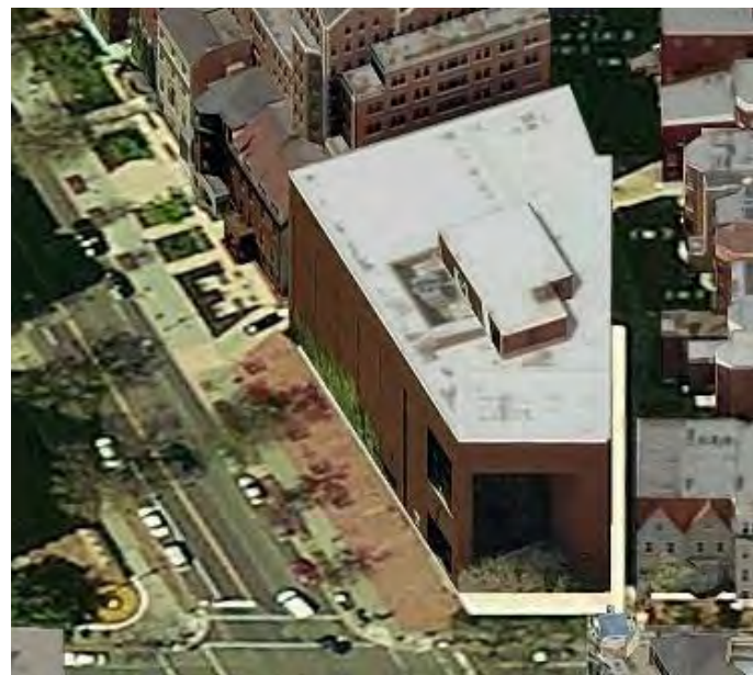
AERIAL VIEW OF EXISTING BUILDING
