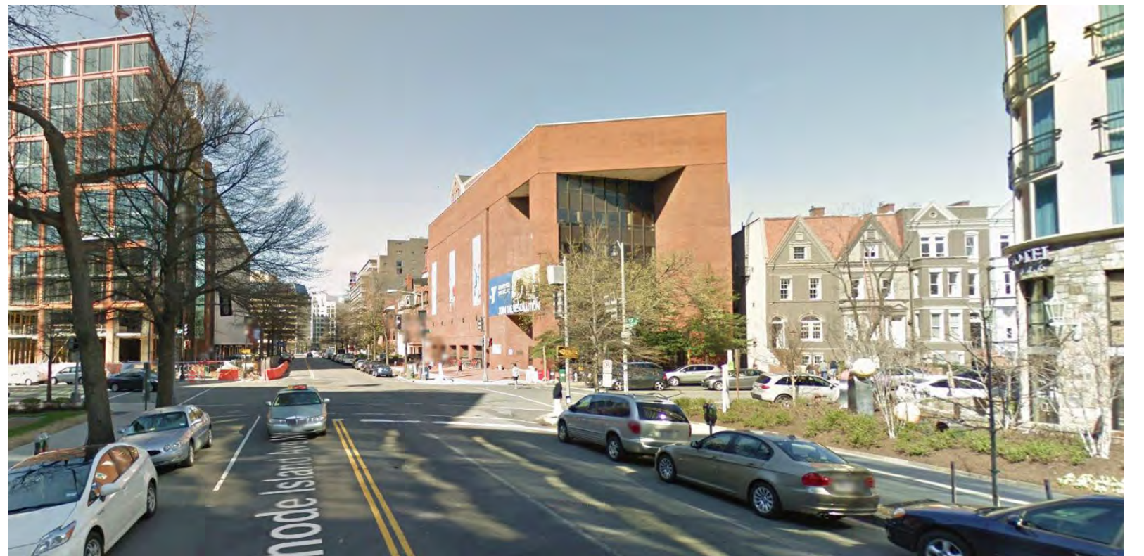
2. VIEW LOOKING WEST, DOWN RHODE ISLAND AVE
