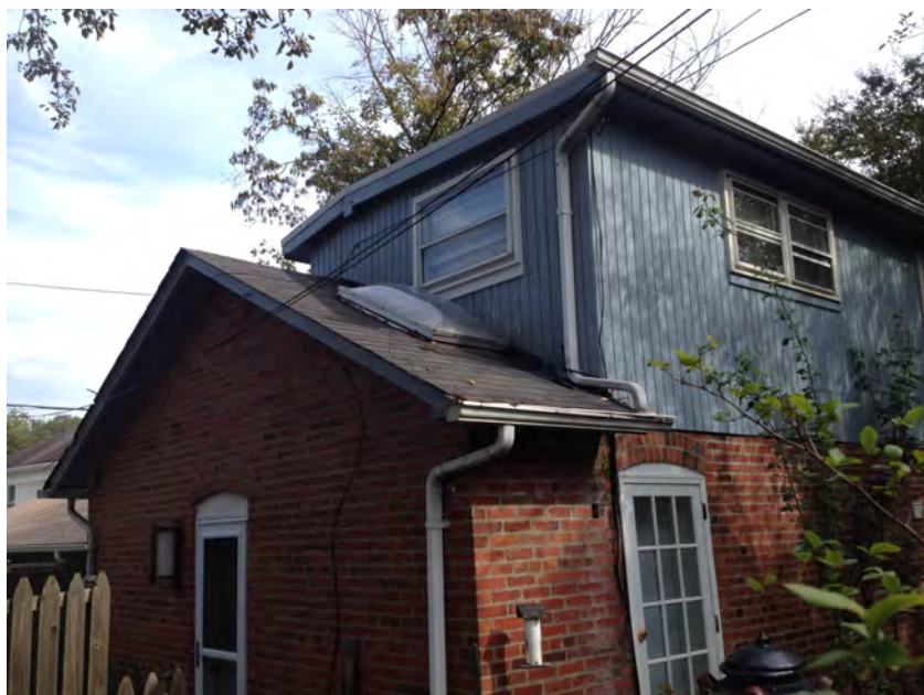
FRONT: EXISTING SECONDARY BUILDN
