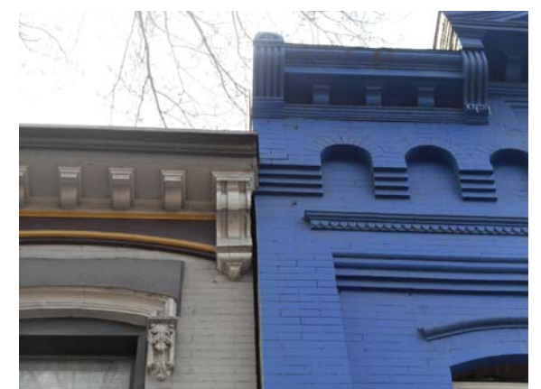
BUILDING @ PROPERTY LINE
