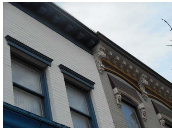
BUILDING @ PROPERTY LINE
