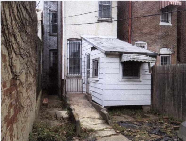
Existing Addition at Rear of Dogleg
