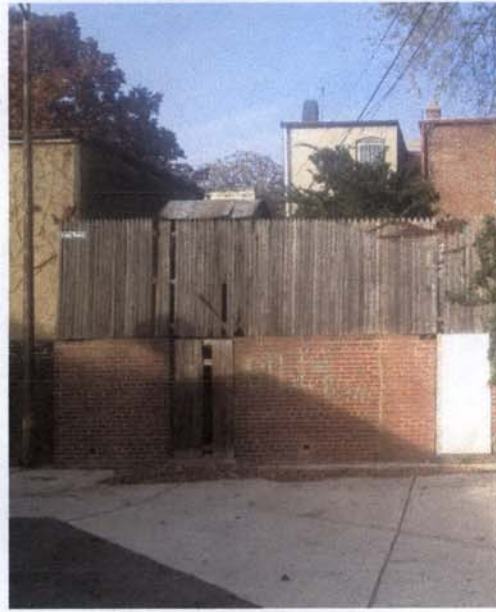
Rear of Property Retaining Wall
