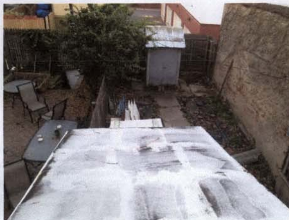
Roof of Existing Addition
