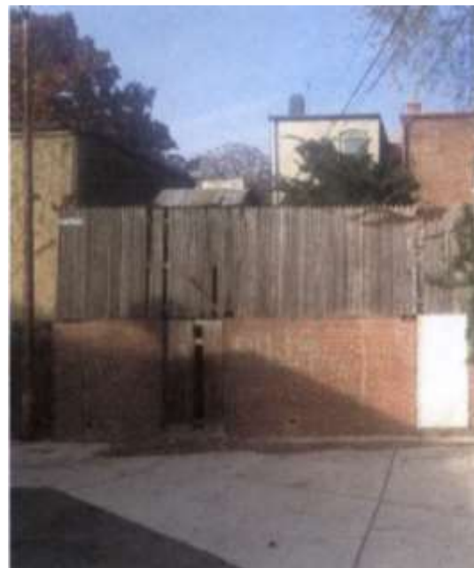
14-foot high wall and fence along the rear property line and abutting the alley.
