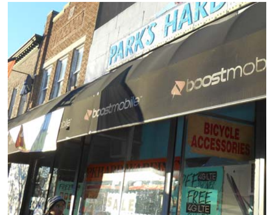
EXISTING FACADE MATERIALS
