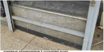
- EXISTING STOREFRONT & MASONRY BASE
