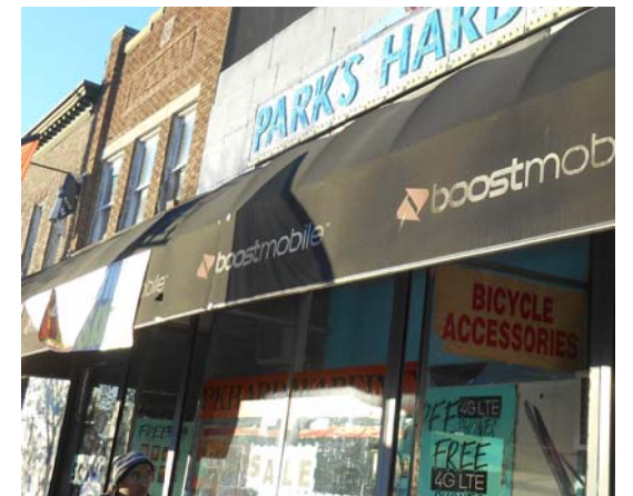
EXISTING FACADE MATERIALS
