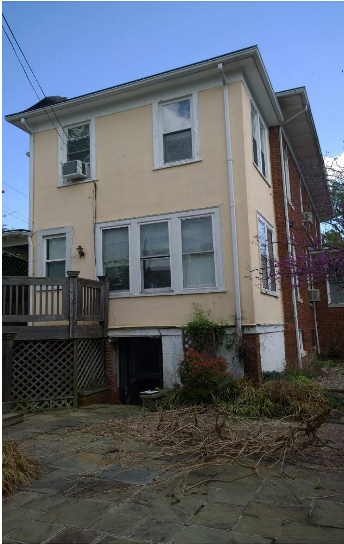
EXISTING REAR VIEW FROM YARD
