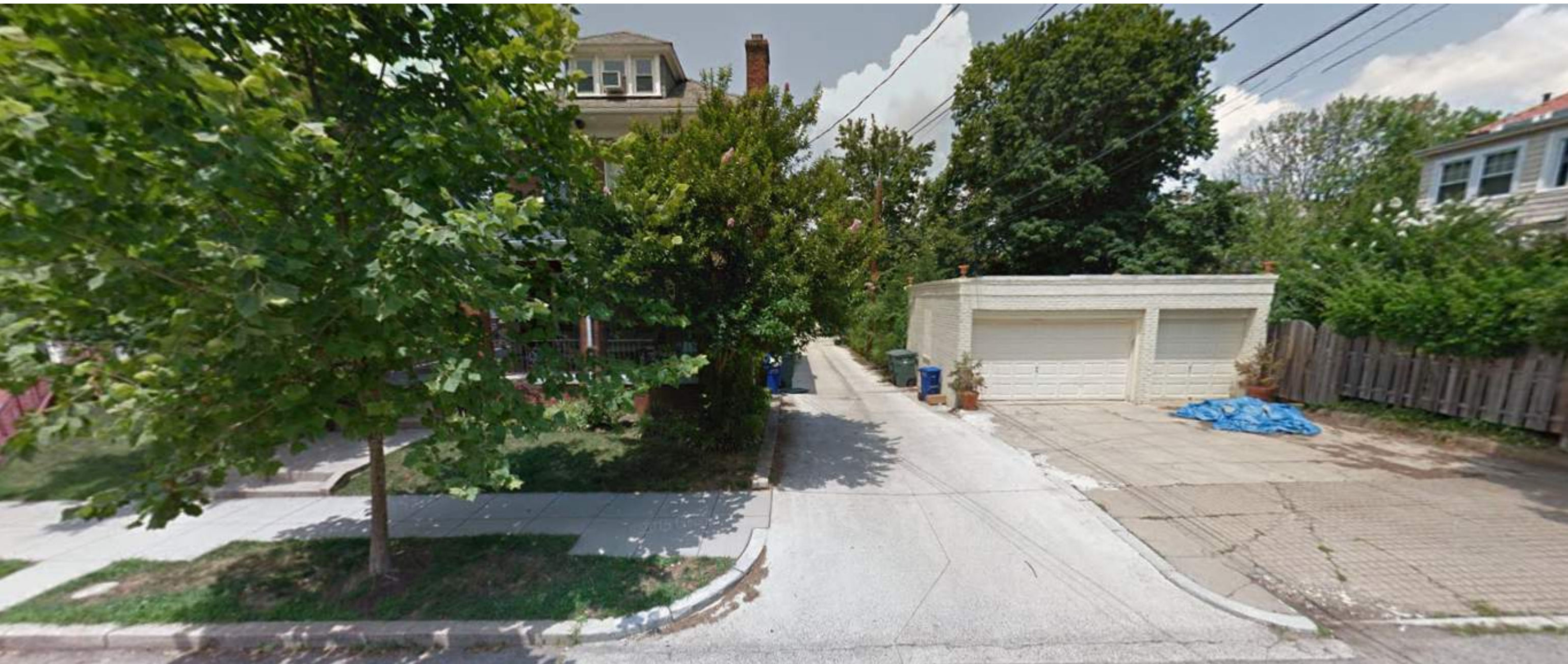
EXISTING ALLEY VIEW ON RIGHT SIDE
