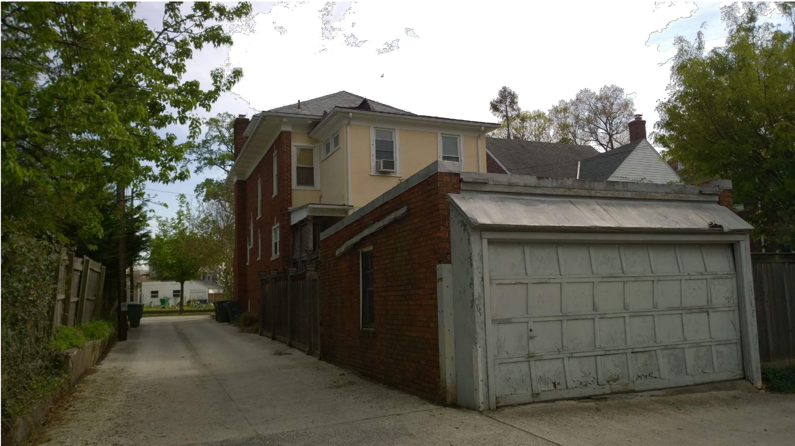
EXISTING REAR VIEW FROM ALLEY
