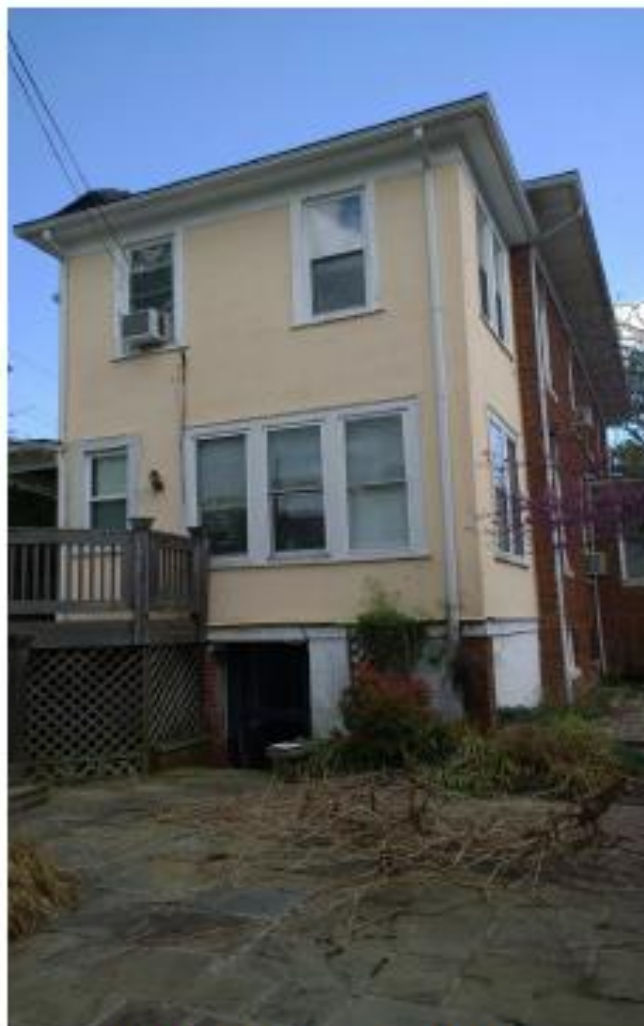
EXISTING REAR VIEW FROM YARD
