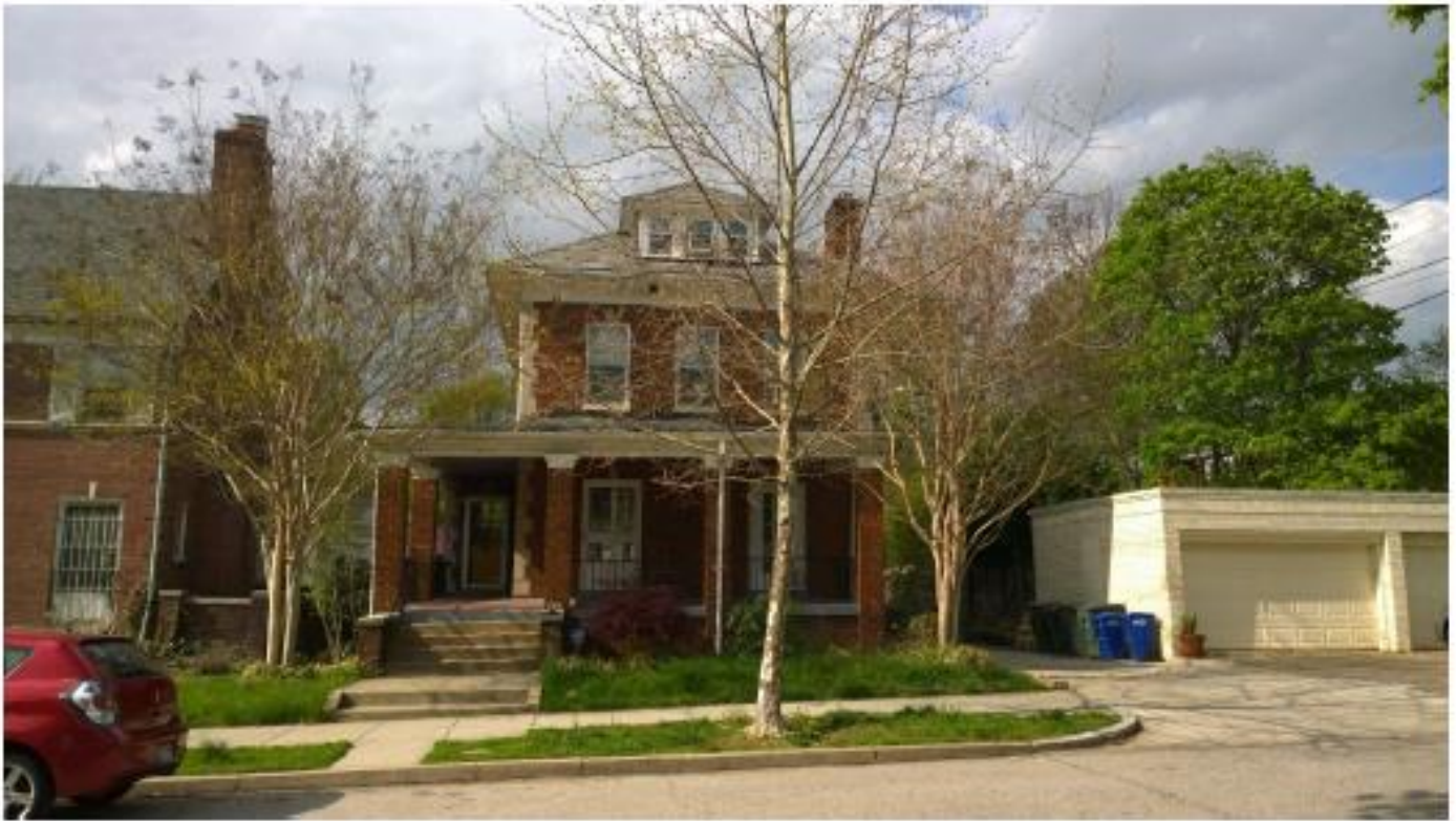
EXISTING FRONT VIEW OF RESIDENCE
