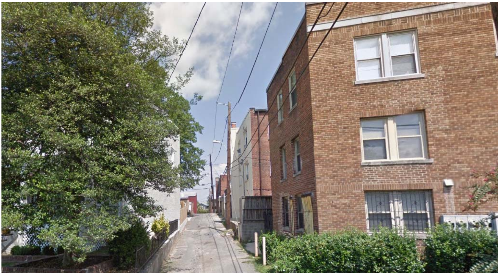
Rear of 4506 Georgia Avenue as seen from Allison Street NW- no parking spaces in the rear
