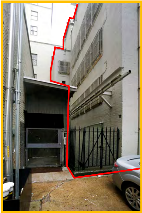
ENLARGED VIEW OF EXISTING NON-COMPLIANT REAR YARD
