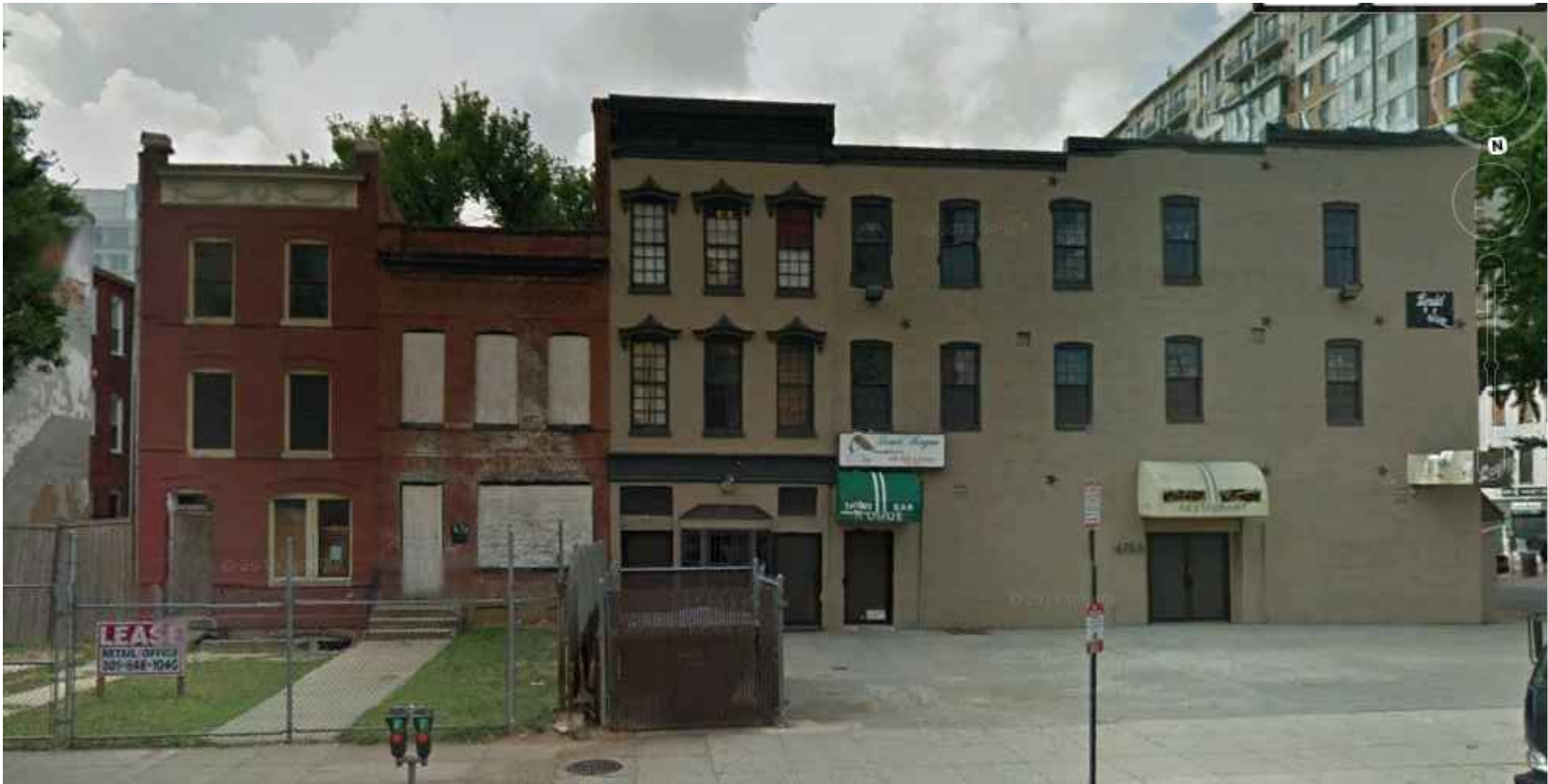
A - VIEW FROM K STREET OF BUILDING PRE-COLLAPSE
