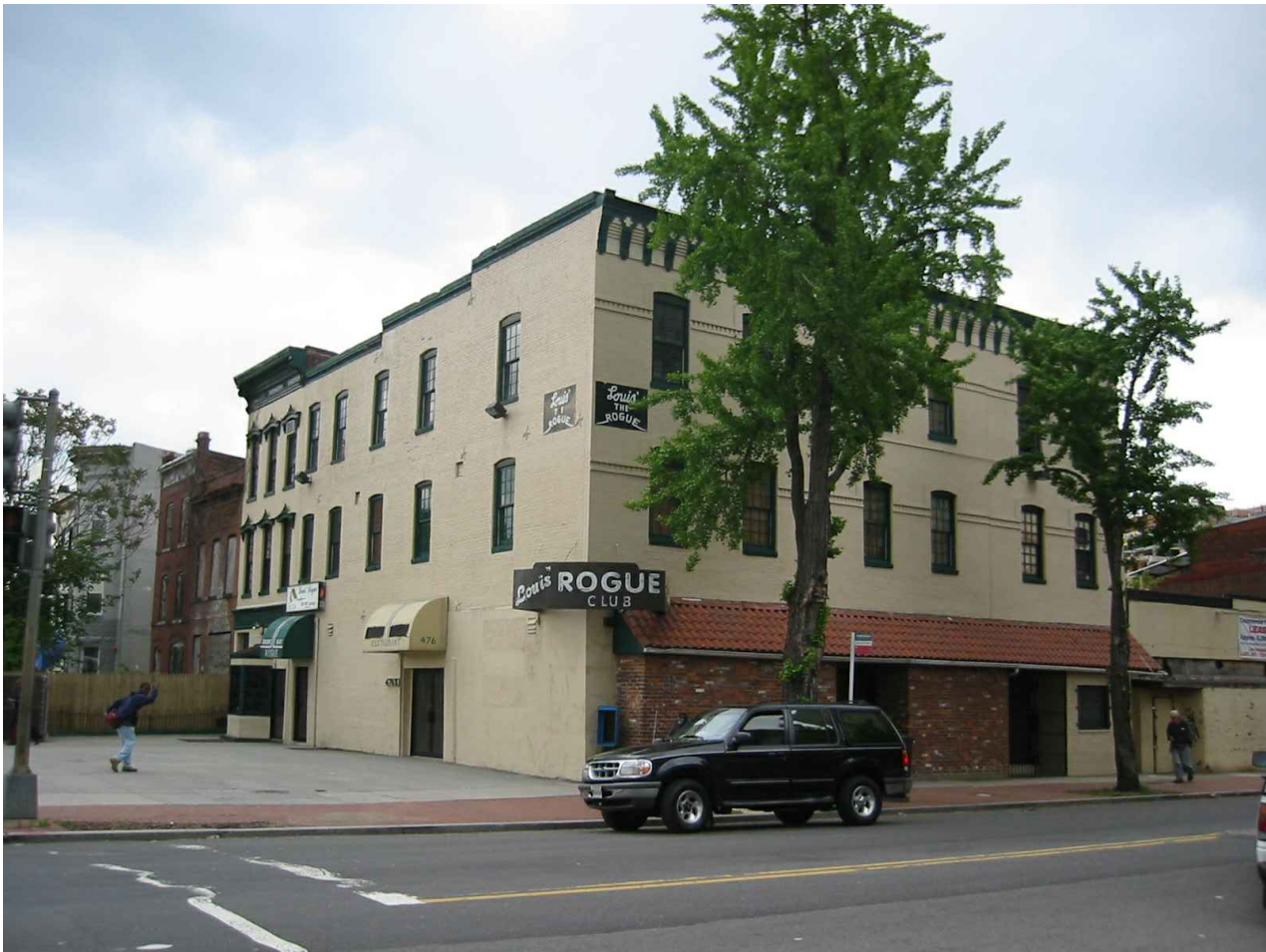
B - VIEW FROM NORTHWEST OF BUILDINGS PRE-COLLAPSE
