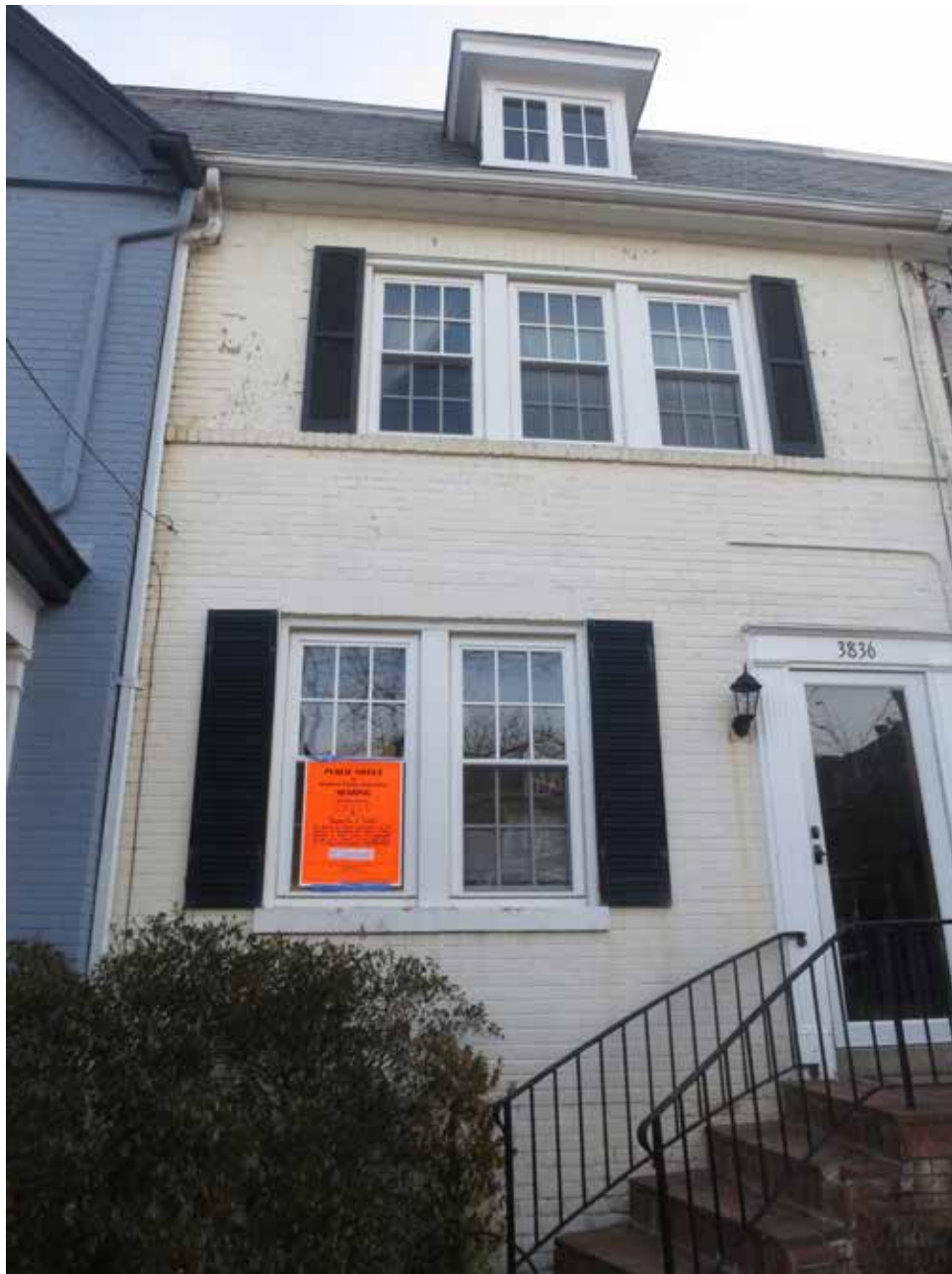
Photo 1—Sign in window 3836 Beecher Street, NW Washington DC 20007
