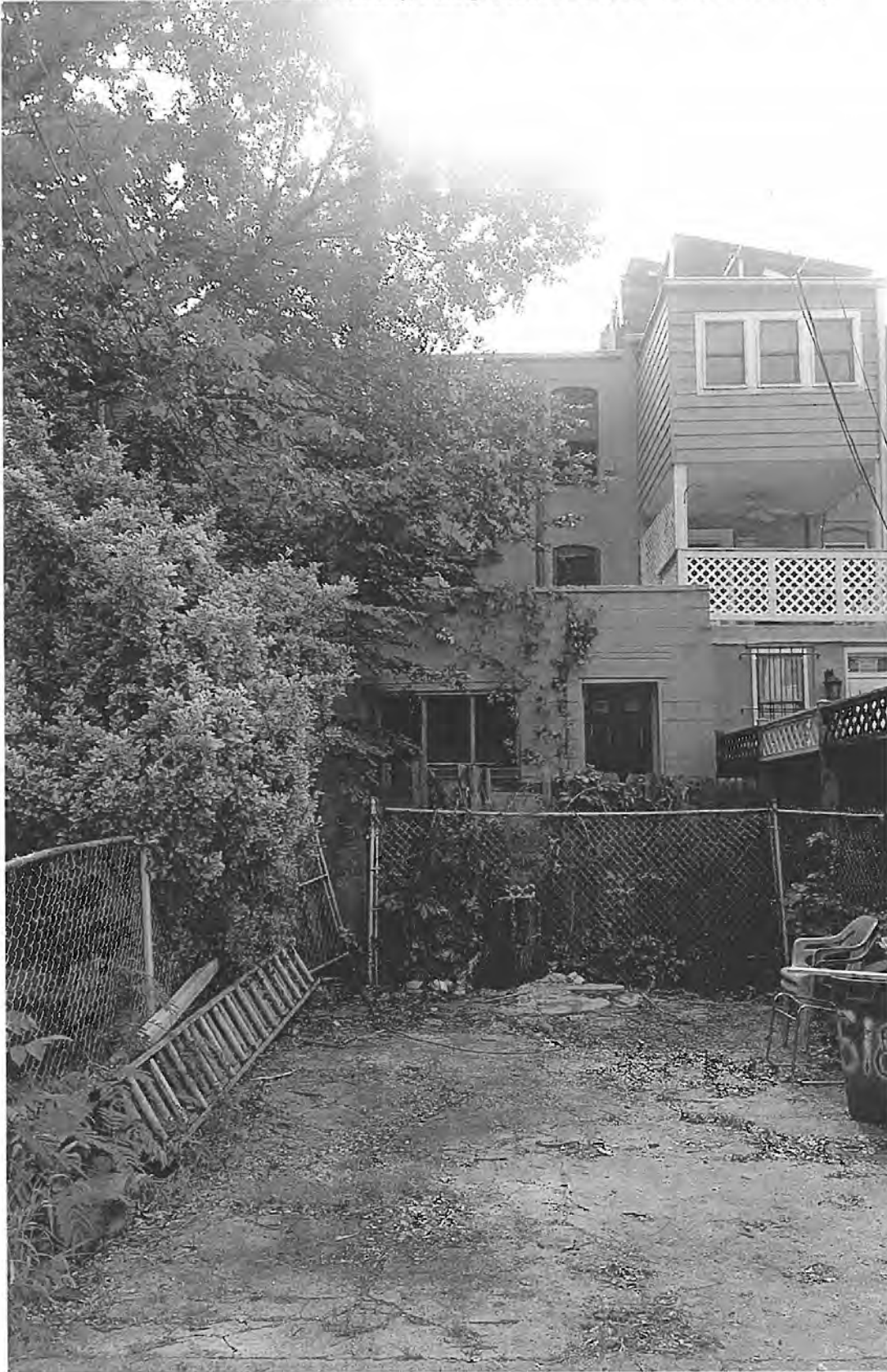
518 6th St., NE (blue house) (rear view from alley, showing no second or third floor over kitchen extension)
