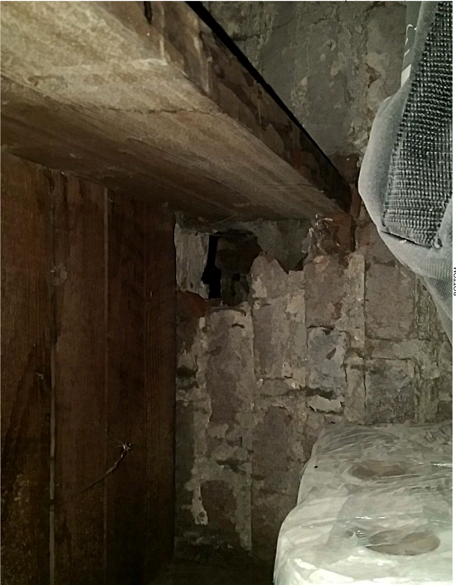
Attachment F - photo of damage to party wall in basement of 520 6th St., NE, caused by work at 518 6th St., NE
