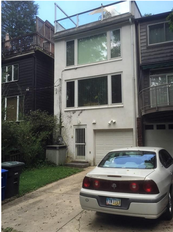
Photos 6. Examples of Sideward Additions on 44 th Street.
