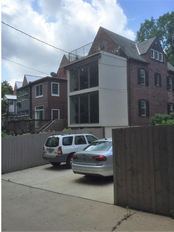
Photos 5. Renovations without decks on 44 th Street Alley
