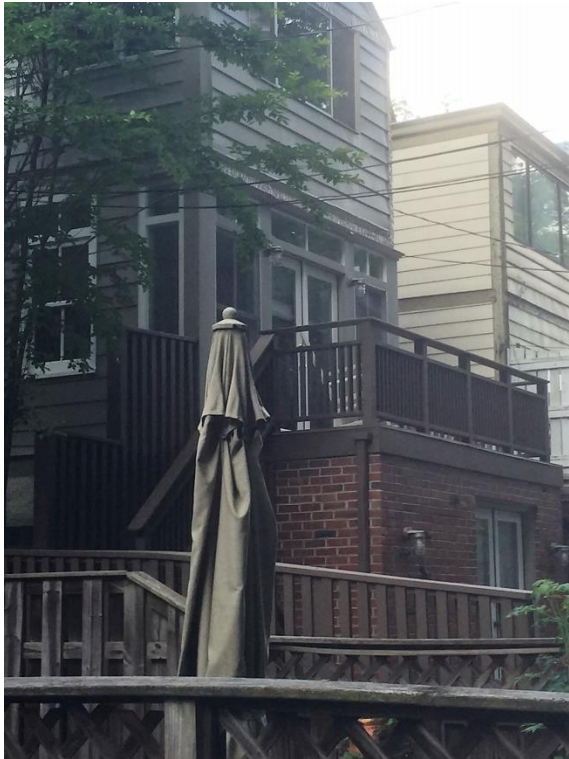
Photo 2. Existing Addition to 1539 already extends approximately 6 feet beyond original façade.
