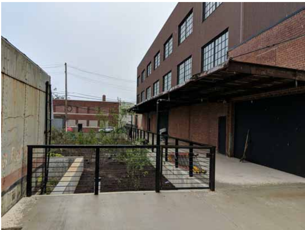
VIEW OF WEST BUILDING FROM TRAINCAR & PLAZA
