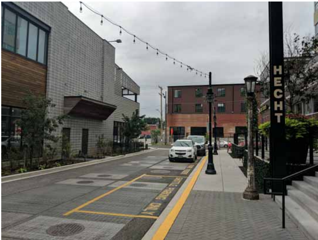
VIEW LOOKING SOUTH FROM HECHT AVENUE NE
