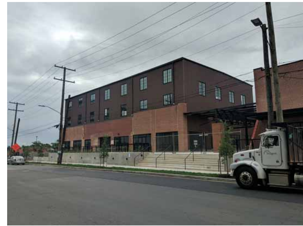
FRONT VIEW LOOKING SOUTHEAST FROM OKIE STREET NE
