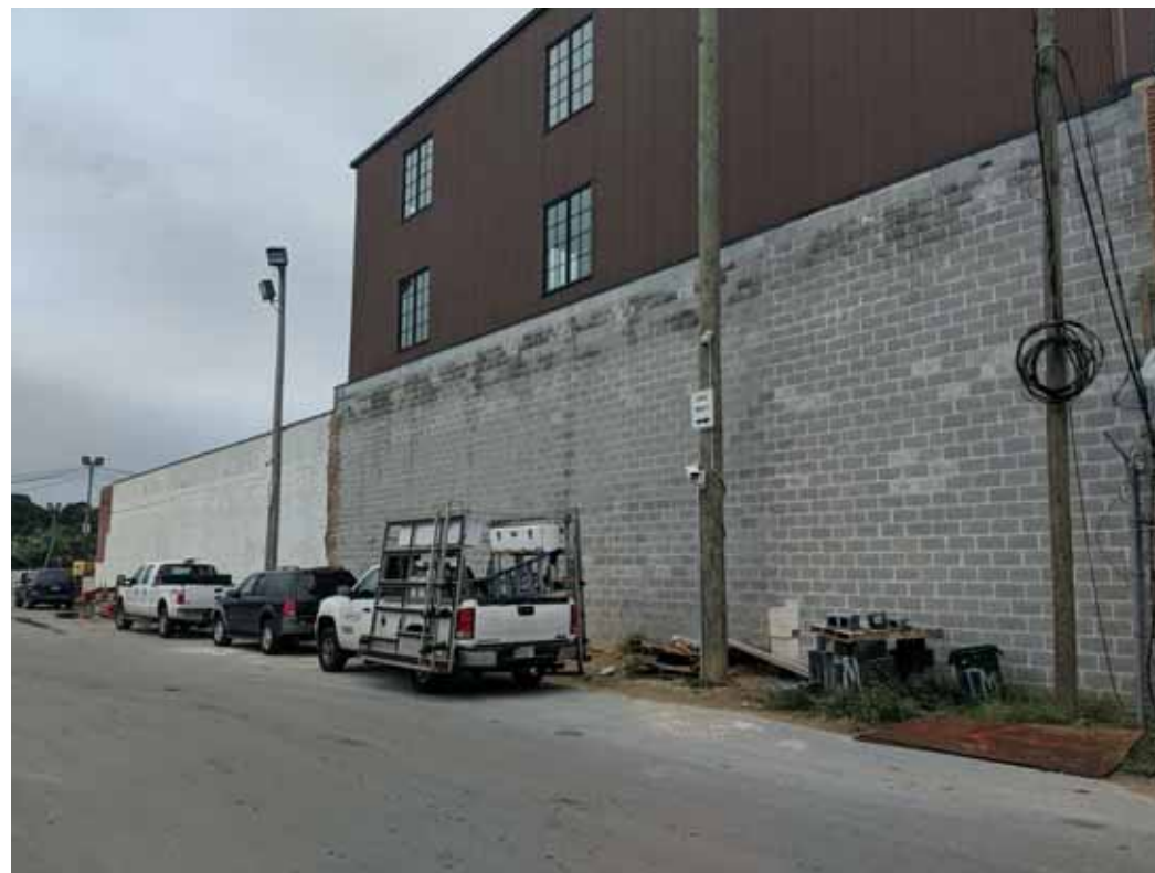
VIEW OF SIDE YARD LOOKING SOUTHWEST FROM OKIE STREET NE
