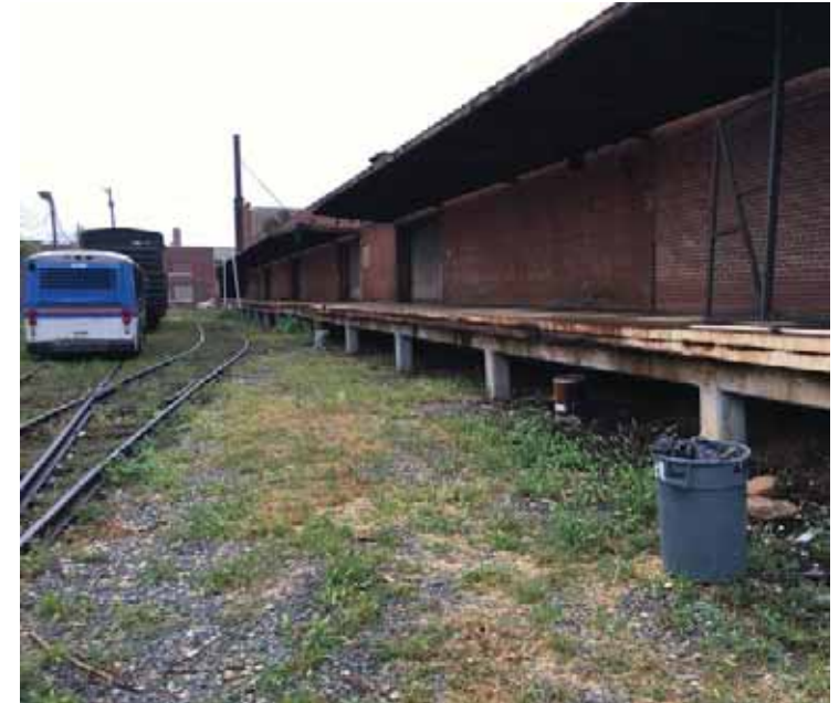
REAR VIEW OF BUILDING LOOKING WEST
