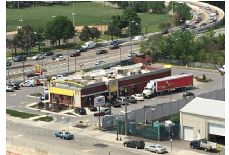
Site Photo 1 - Aerial looking NW
