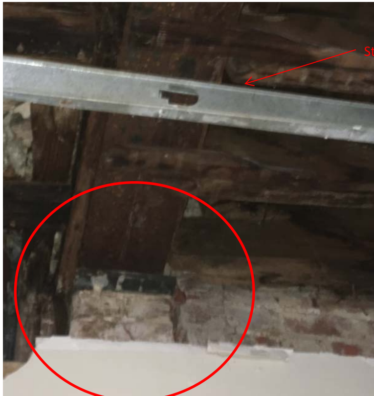
Below Second Floor Window, Steel Beam and Structural Issues with Brick
