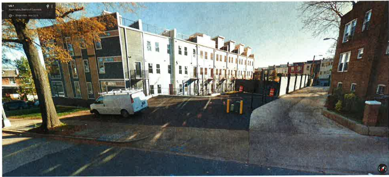
Figure 2: Photo of Curb Cut and Public Space on Rhode Island Avenue for Lots 42 and 43 (Source: Google Maps)
