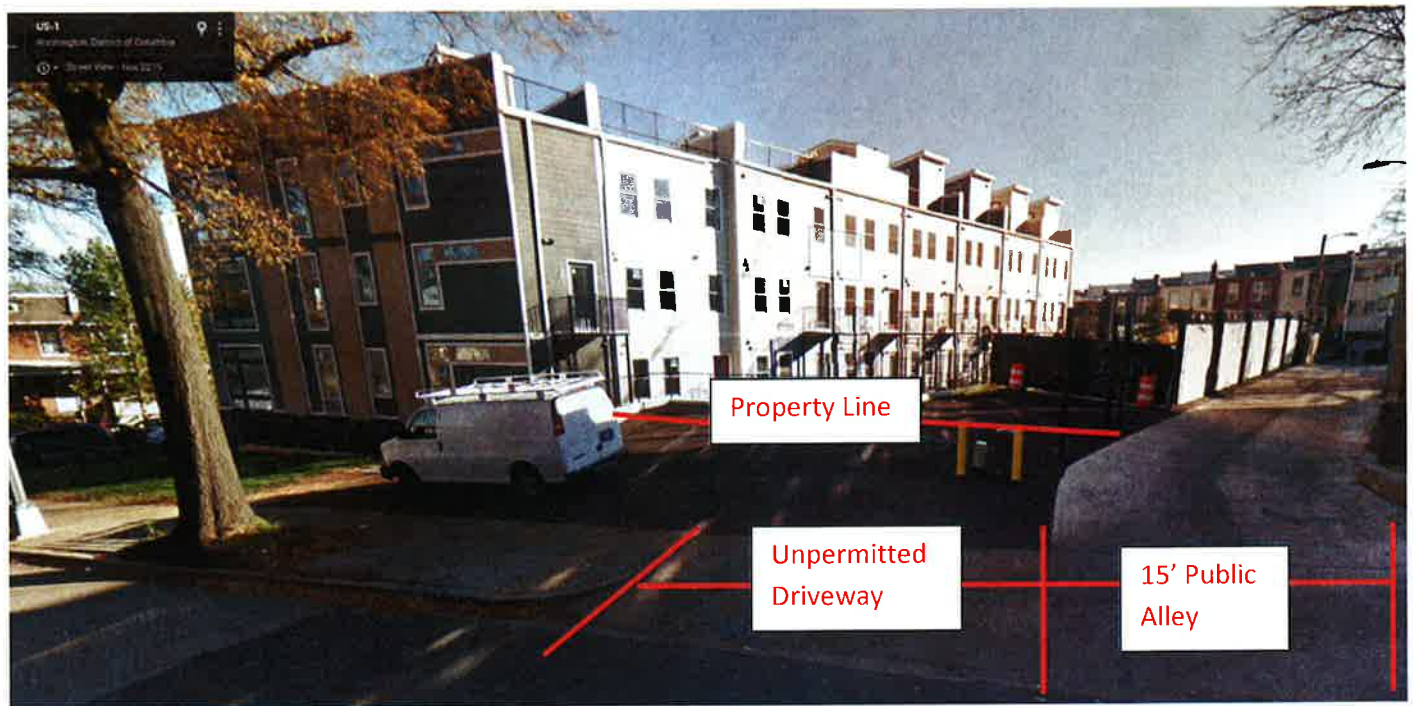
Figure 2: Photo of Curb Cut and Public Space on Rhode Island Avenue for Lots 42 and 43 (Source: Google Maps)
