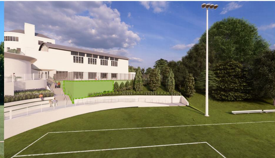
NEW RETAINING WALL TO SUPPORT PRACTICE FIELD (13.6' MAX)
