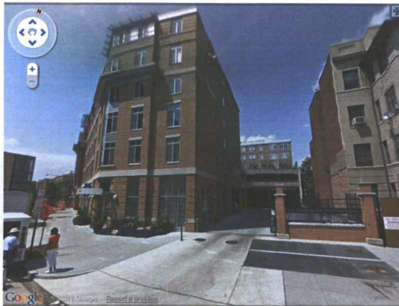
View of area for addition from Kenyon Street.
