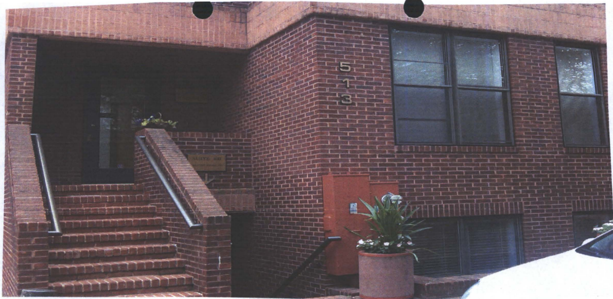
513 Capitol Court Suite 200 NE Front Entrance
