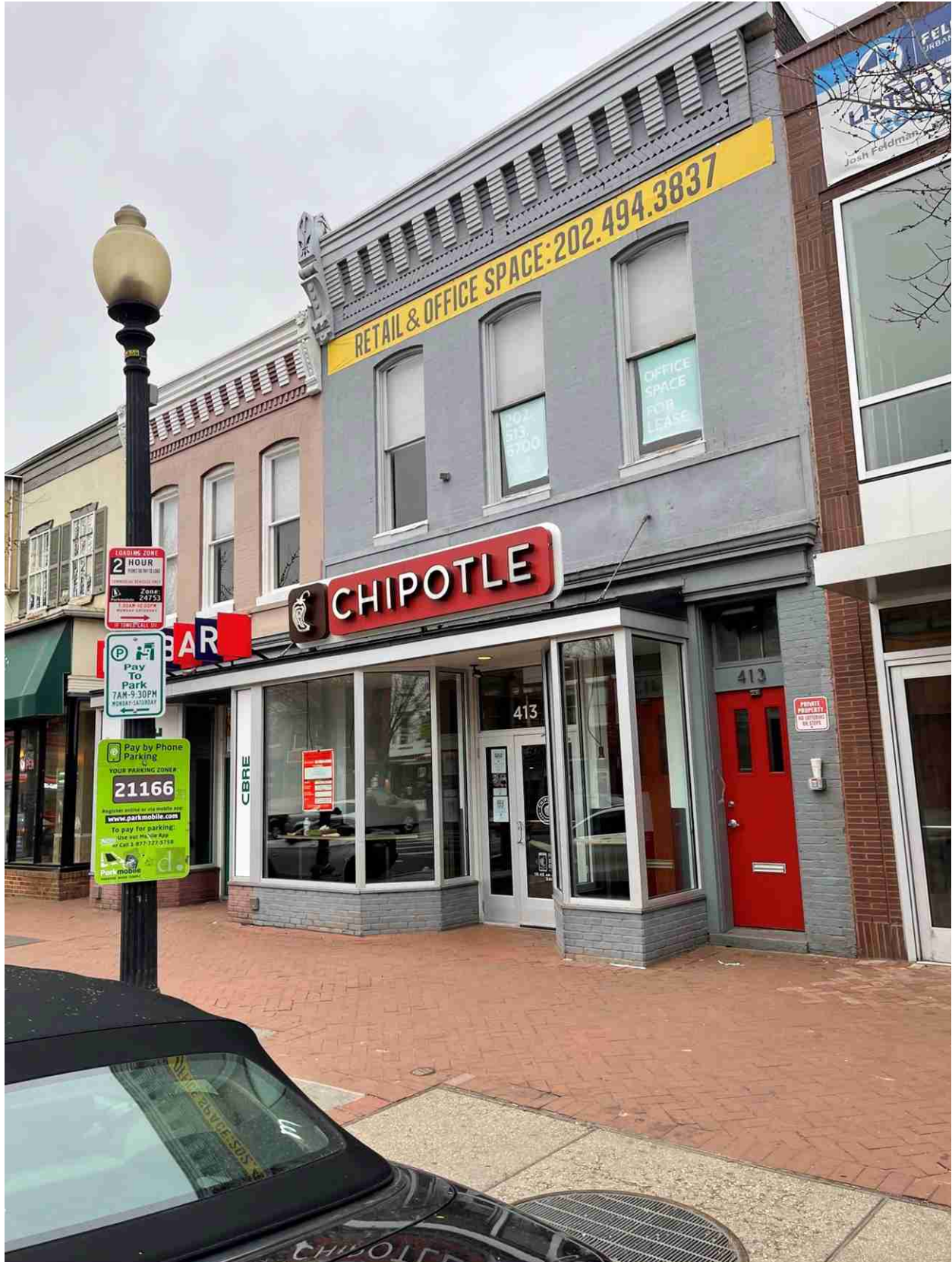
Application Case No. 18238A Color Photographs of 413 8 th St., SE, Washington DC, 20003
