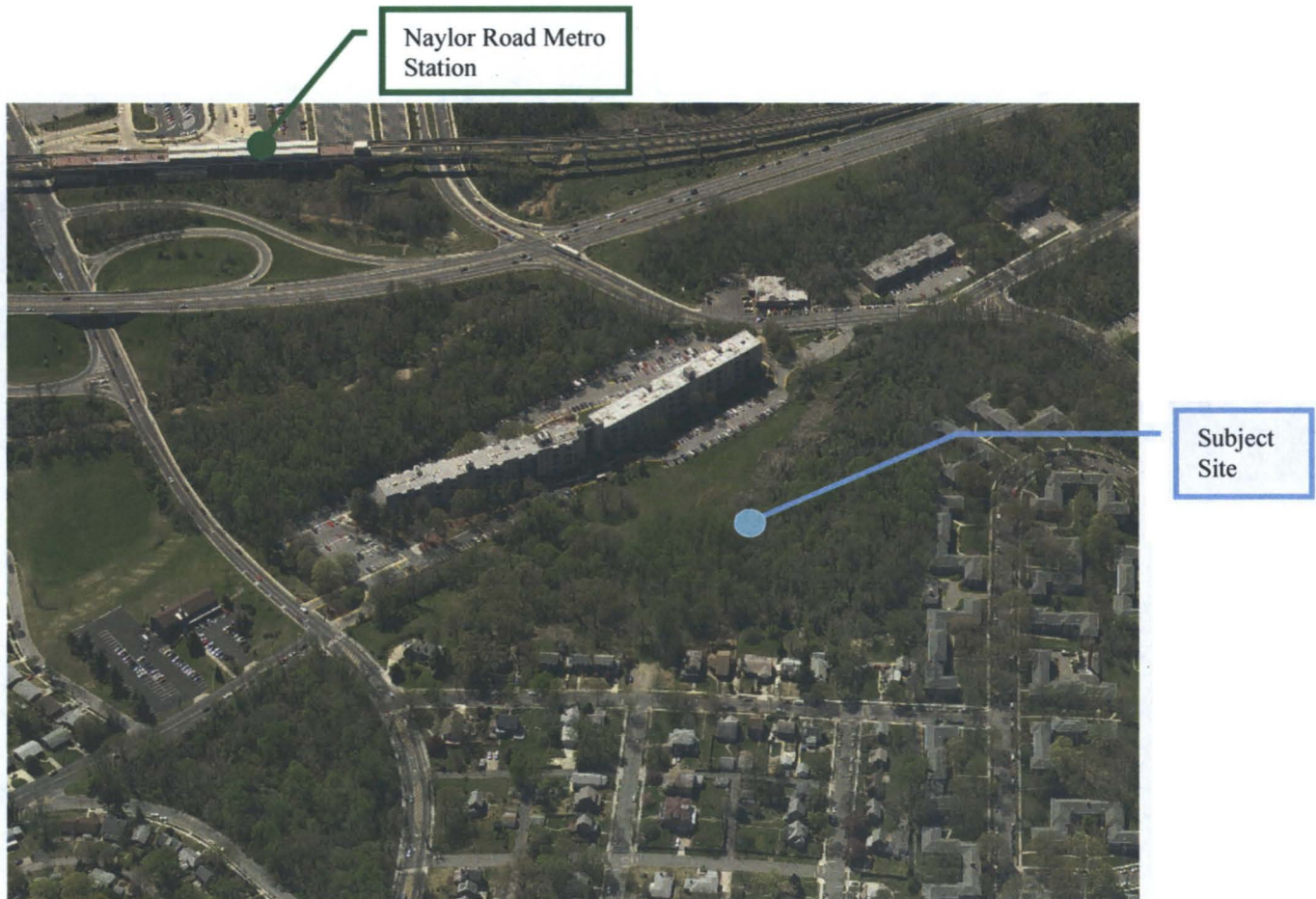
Aerial view from the west looking toward the Maryland border
