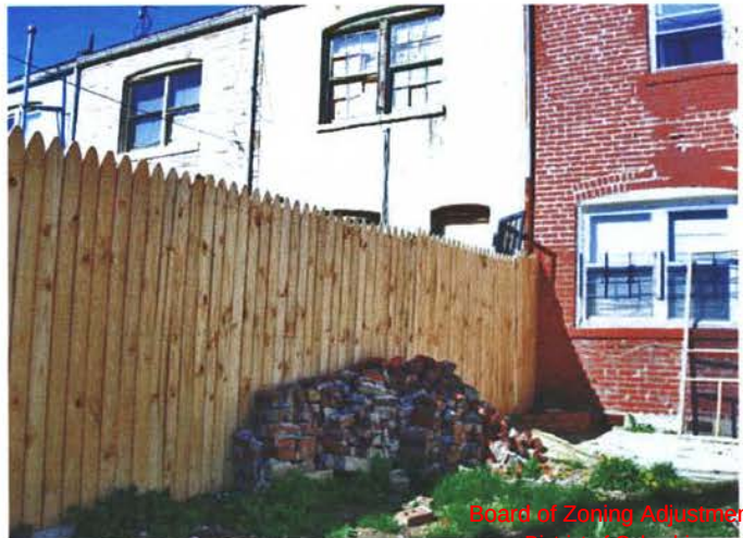
North Alley View
