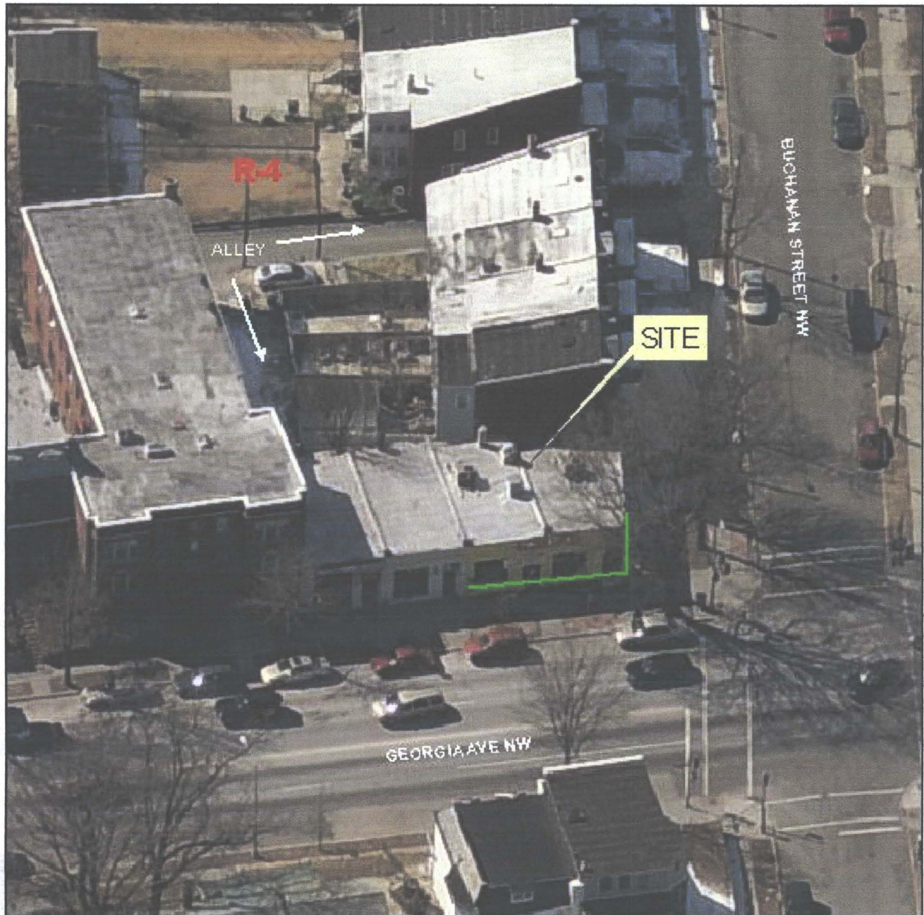
BZA Application No. 17801 View to the West
