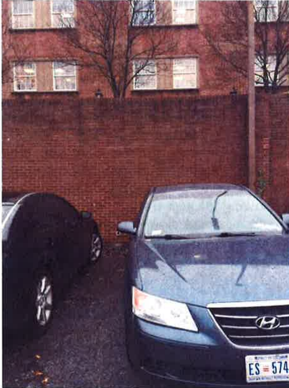
Image 1 Post Office Retaining Wall
