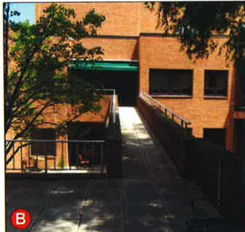
View of Existing Bridge Looking From Tennis Courts Towards Washington Home
