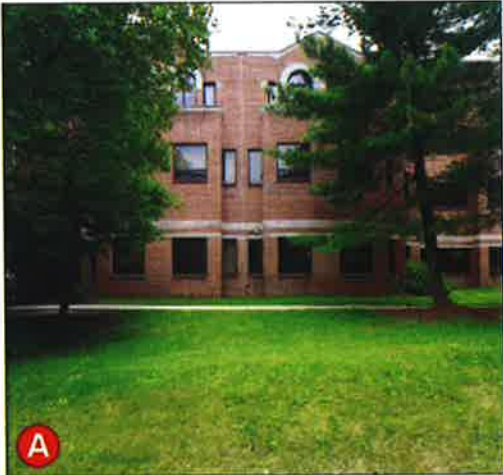
Close Up View of Existing Facade
