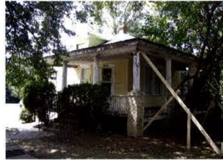
5 HOUSE AT 6924 WILLOW STREET TO BE RELOCATED
