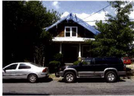
4 HOUSE AT 6926 WILLOW STREET TO BE RECONSTRUCTED
