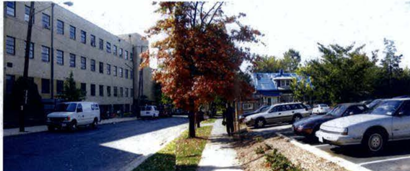
8 WILLOW STREET LOOKING SOUTH
