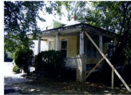
5 HOUSE AT 6924 WILLOW STREET TO BE RELOCATED
