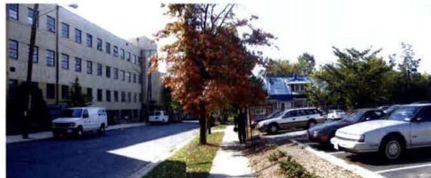
8 WILLOW STREET LOOKING SOUTH
