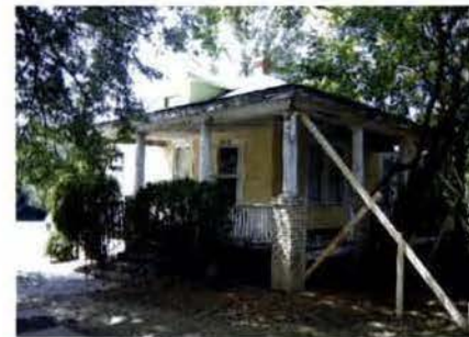
5 HOUSE AT 6924 WILLOW STREET TO BE RELOCATED
