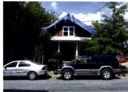
4 HOUSE AT 6926 WILLOW STREET TO BE RELOCATED
