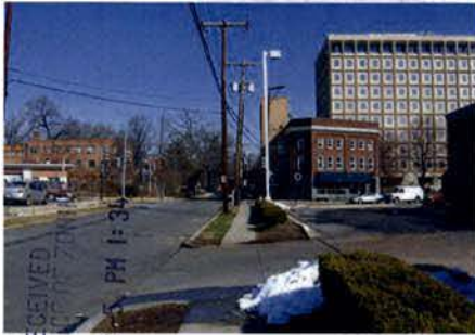
3 MAPLE STREET LOOKING NORTH
