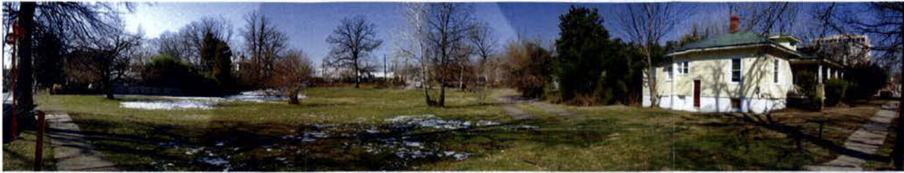
① EXISTING SITE ALONG WILLOW STREET
